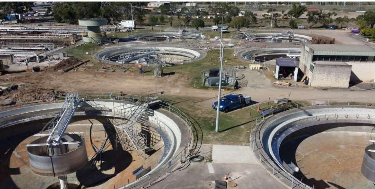
*“Hydroflux can provide new clarifier internals and refurbish existing systems regardless of the clarifier tank design and geometry”*
